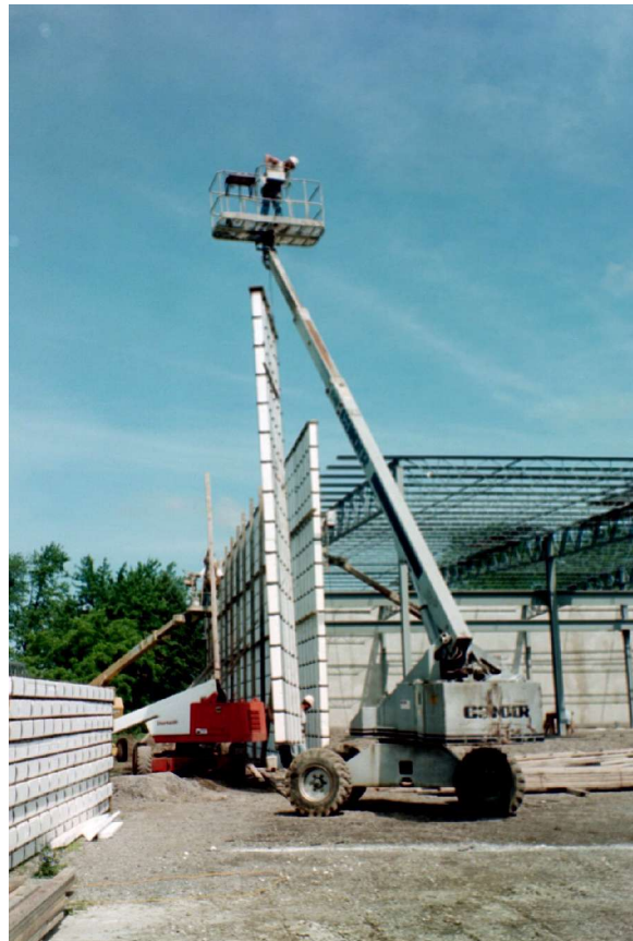
Erection of lightweight wall panels
