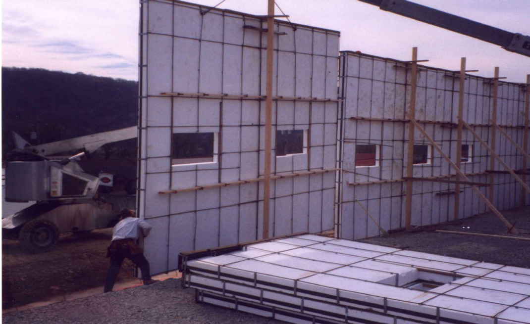
Setting panels on footers
