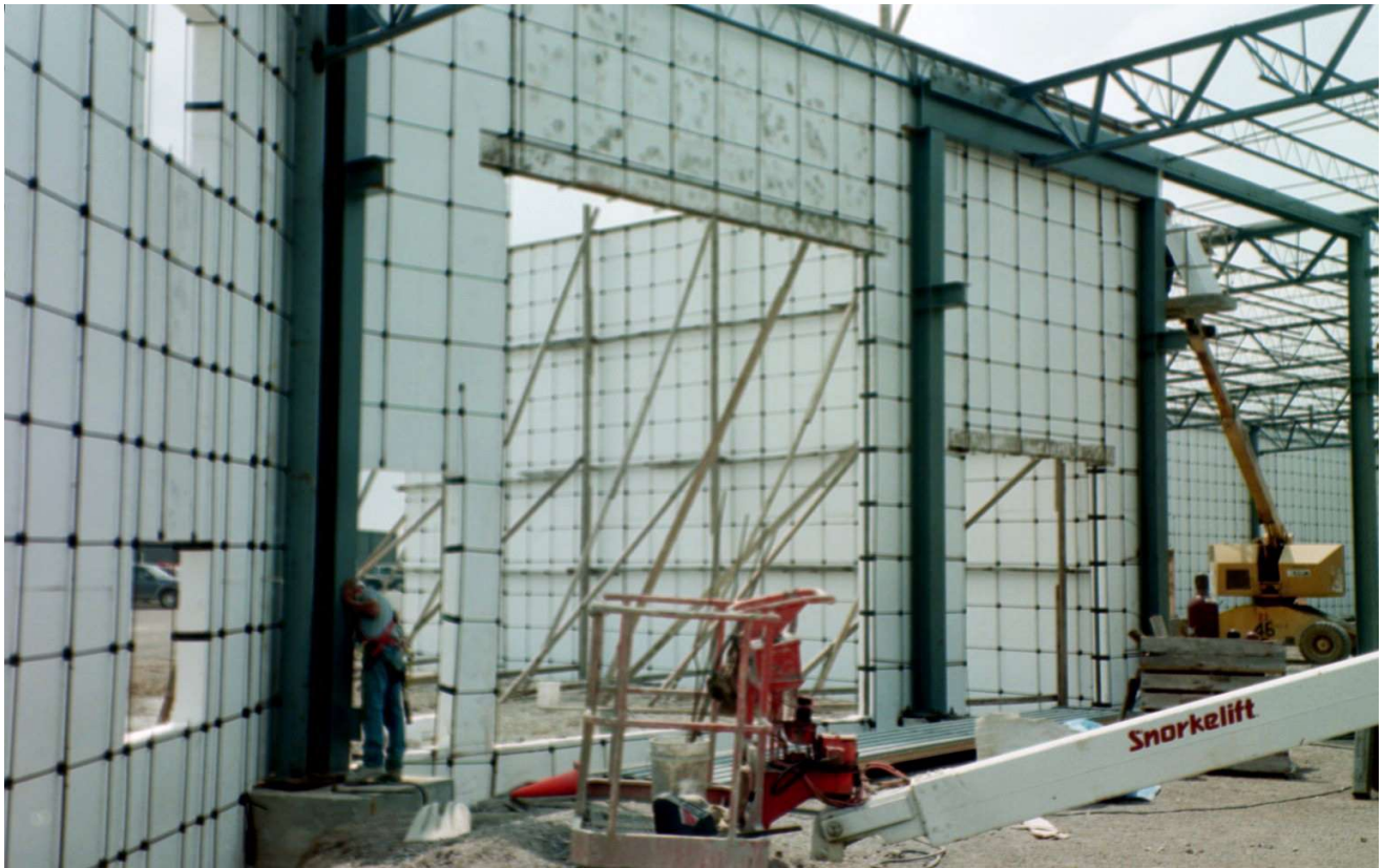
Interface of panels with structural steel
