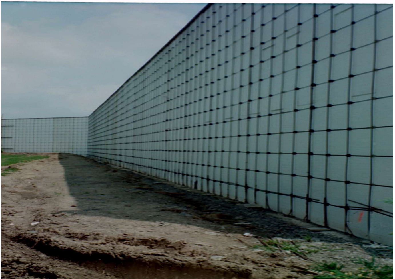
Wall ready for Shotcrete
