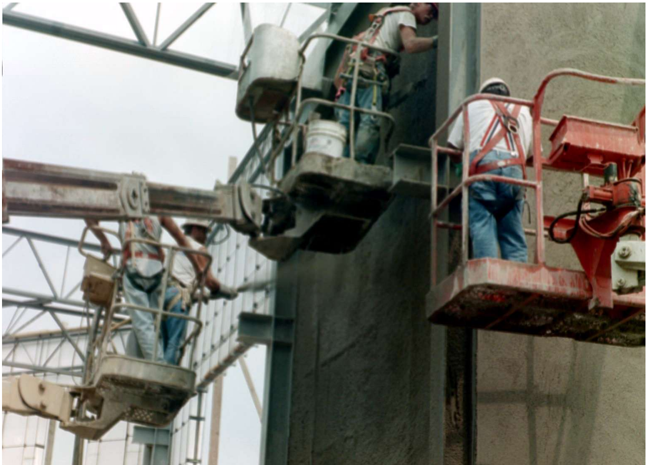
Shotcreting, screeding and finishing the walls
