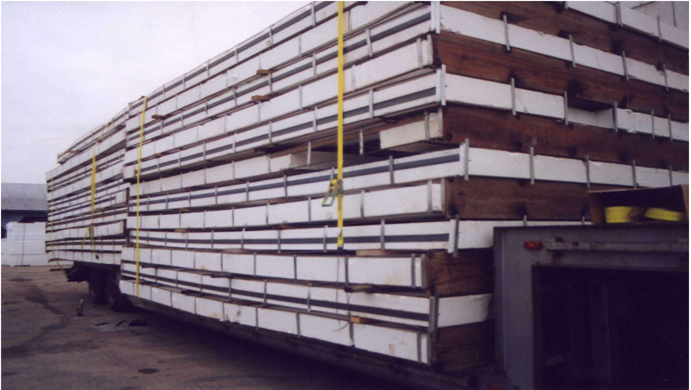
Load of wall panels delivered to jobsite
